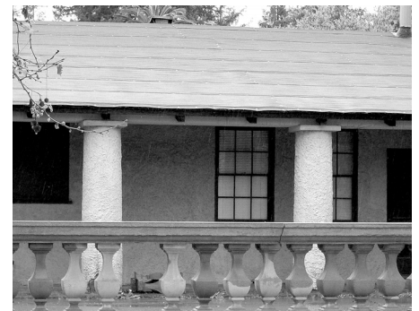
New roof protects East Cottage on a rainy day.
